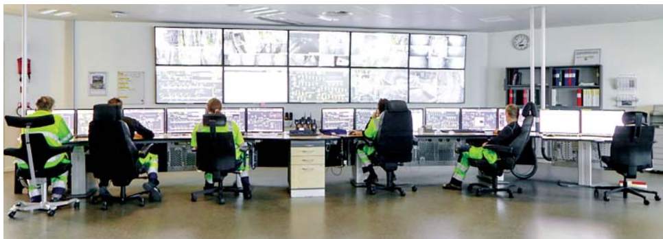
The ventilation control room at Boliden's Garpenberg mine. (Photo: ABB)
